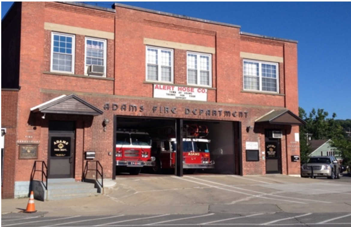
Figure II-2 Adams Fire District Headquarters 3 Columbia Street Adams Mass
