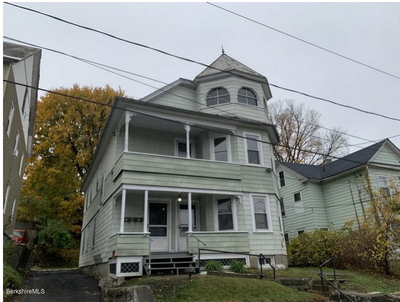
Figure II-17 Balloon Frame Residential Structure Adams, Mass
