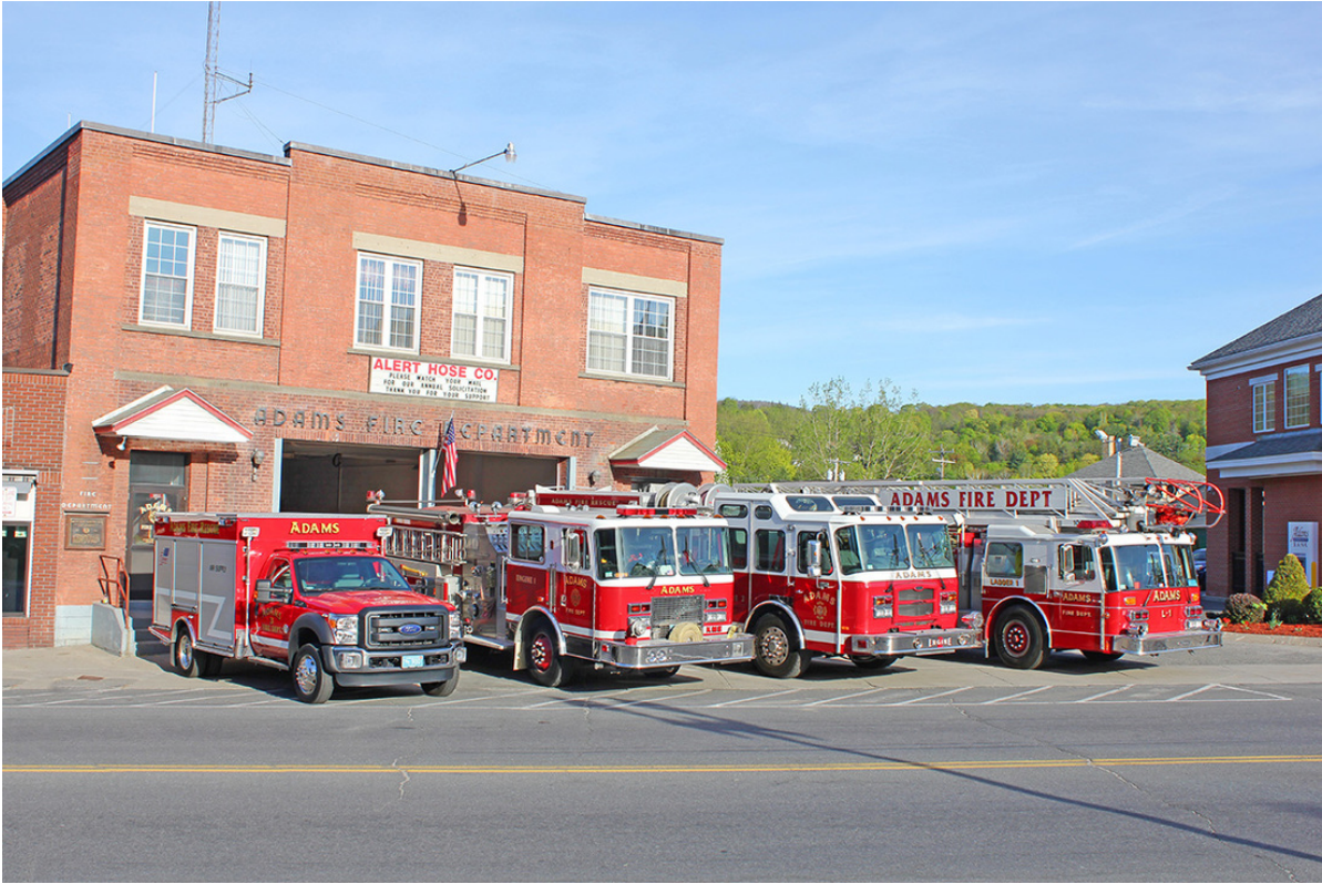
Figure II-3 Adams Fire District Fire Department Apparatus
