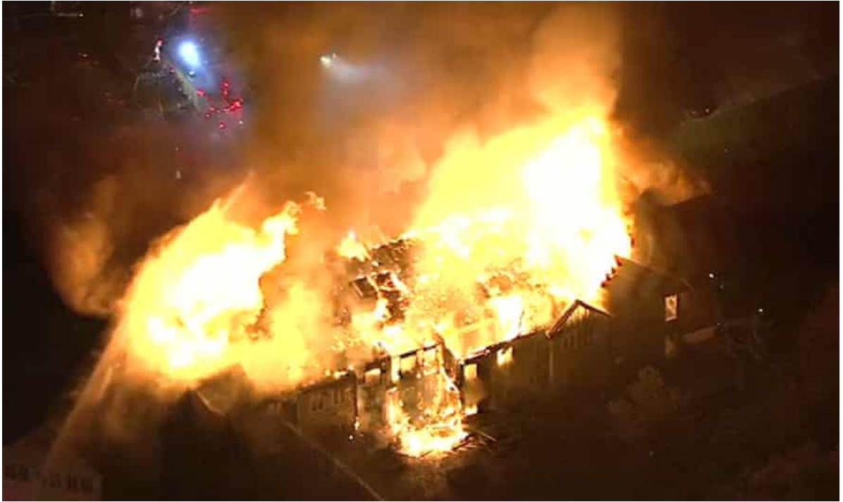
Figure II-20 Fire at Barclay Friends Senior Living Facility Wester Chester, PA
